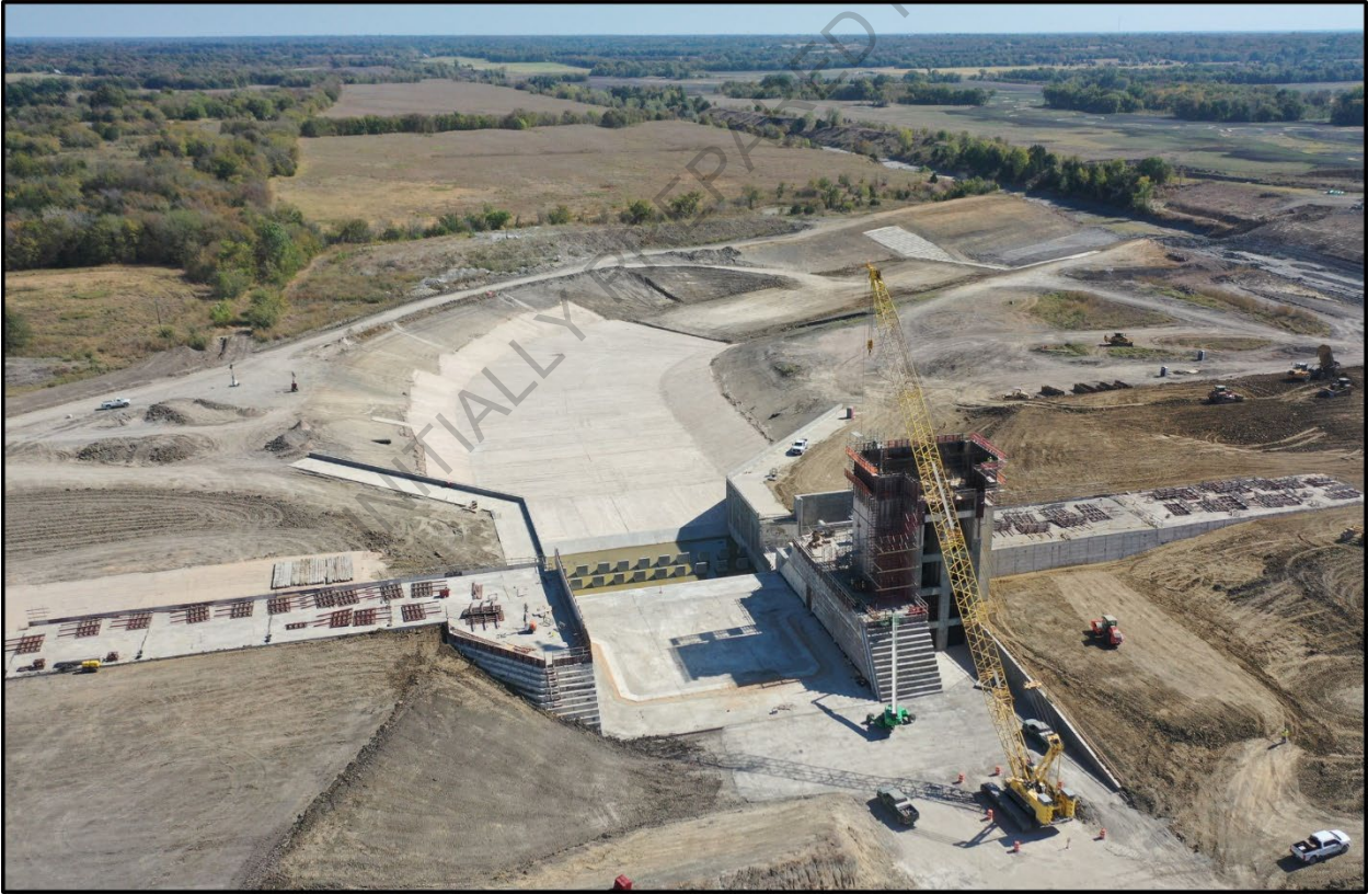
Lake Ralph Hall Spillway Construction
