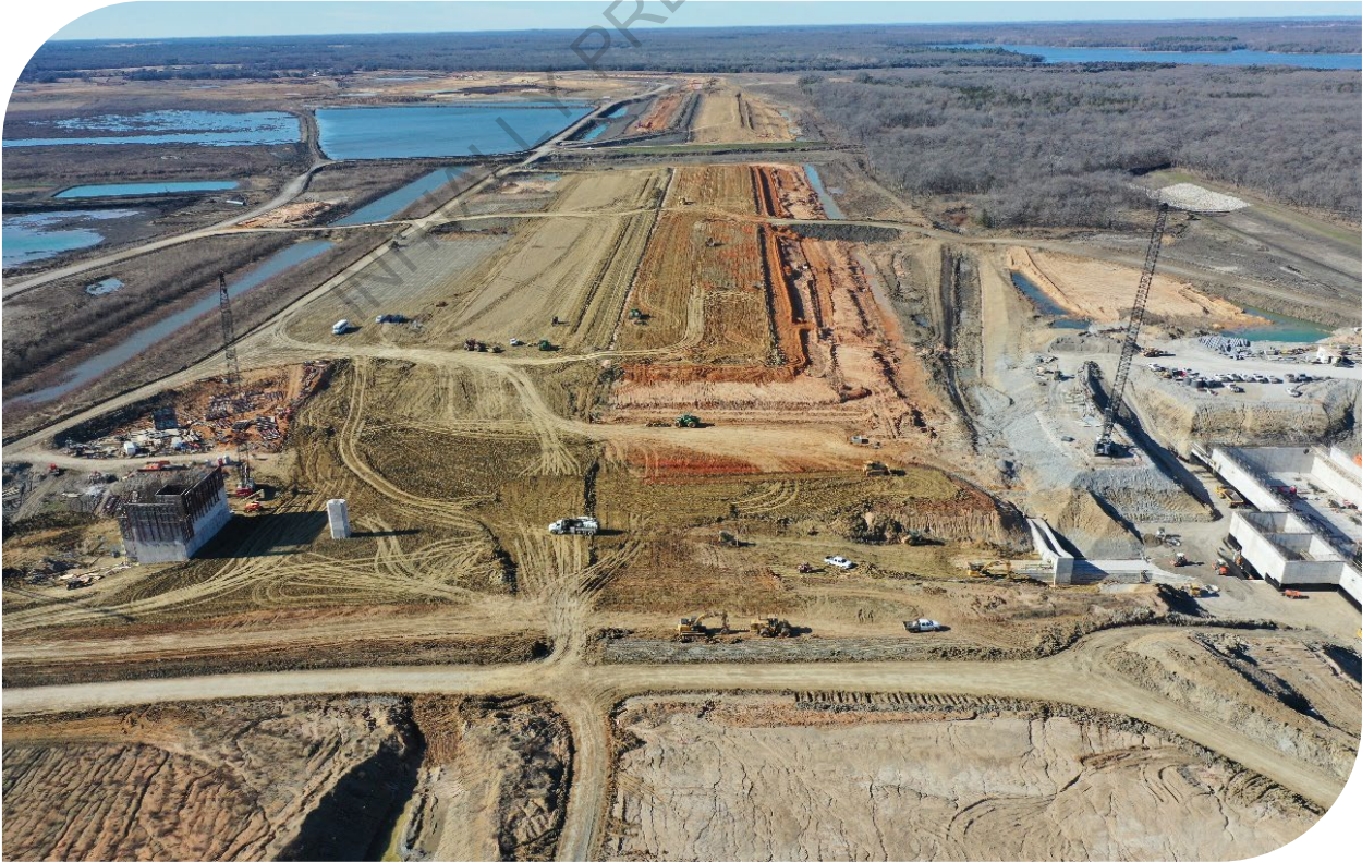
BOIS D'ARC LAKE CONSTRUCTION AERIAL
