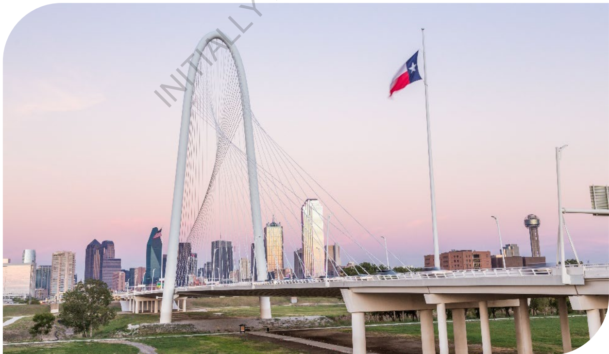
MARGARET HUNT HILL BRIDGE IN DALLAS
