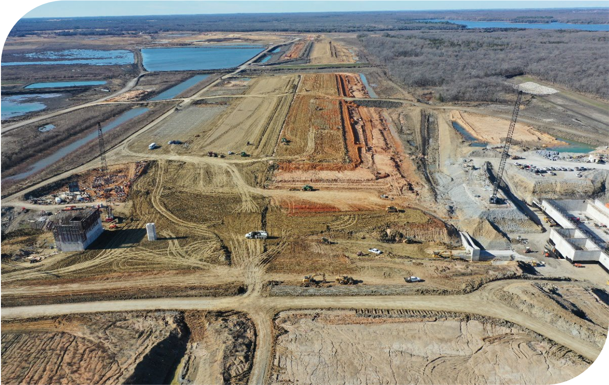
BOIS D'ARC LAKE CONSTRUCTION AERIAL
