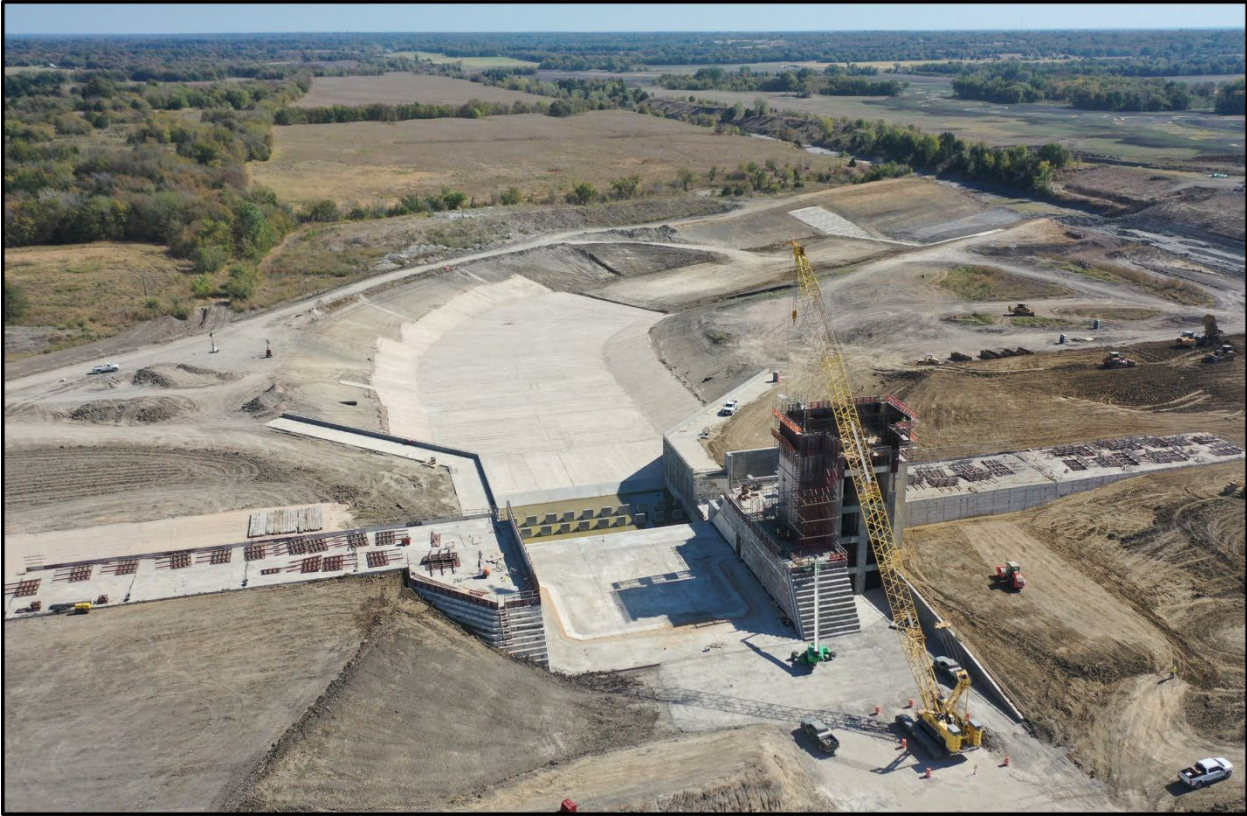
Lake Ralph Hall Spillway Construction
