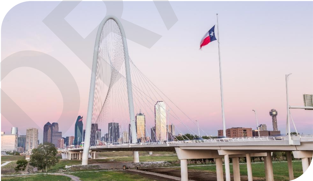
MARGARET HUNT HILL BRIDGE IN DALLAS
